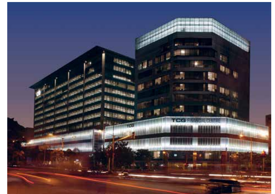
view from across bkc road - fifc on the left with tgc financial centre on right
