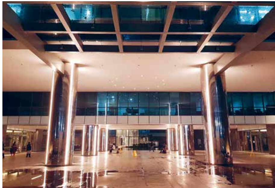
entrance lobby with 8 meter long linear fixtures built-into the columns
